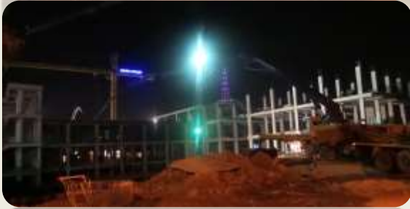
CONSTRUCTION WORK OF DUHOK FAMILY MALL EXTANTION-DARIN GROUP
