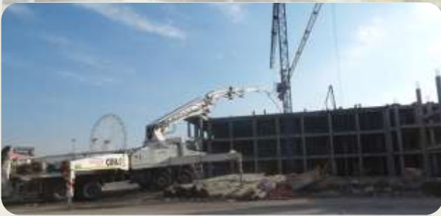
CONSTRUCTION WORK OF DUHOK FAMILY MALL EXTANTION-DARIN GROUP
