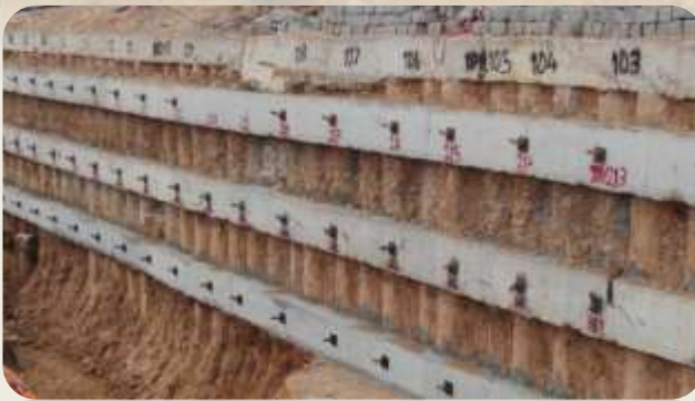
CONSTRUCTION WORK OF EXCAVATION & BEAMS
