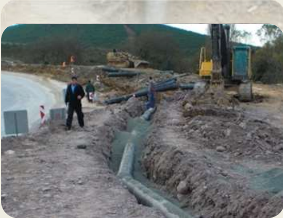
CONSTRUCTION WORK OF İSTANBUL- WIDE NEW ROADS AND ROAD EXTENSIONS
